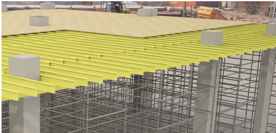
Scaffolding at a construction site
